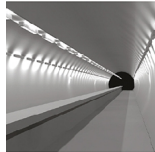
We can provide lighting schemes for tunnels
